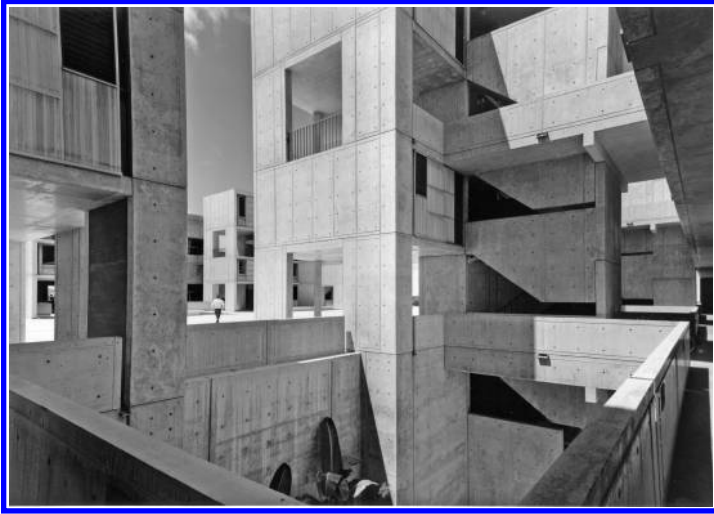
FIG. 8 Ezra Stoller's photograph perfectly captures the complexity of Kahn's design. Note how light and shadow play across the beautifully finished concrete, with its symmetrical plugs. The teak shutters of the studies contrast with the smooth concrete beside them. The light well in the center opens the basement laboratory to the sun. Source: Ezra Stoller, Esto Photographics Inc.
