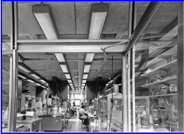
FIG. 7 Kahn's structural innovations opened up the laboratories to football field dimensions. The interstitial space above allowed quick change out and an endless variety of laboratory designs. For the most part, the scientists arranged their labs conventionally, with services at the center and benches around the perimeter. Source: Ezra Stoller, Esto Photographics Inc.
